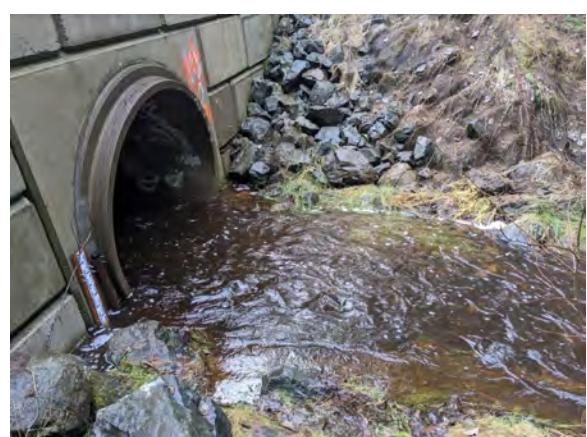
December 26, 2022 / High Flow Section Control
