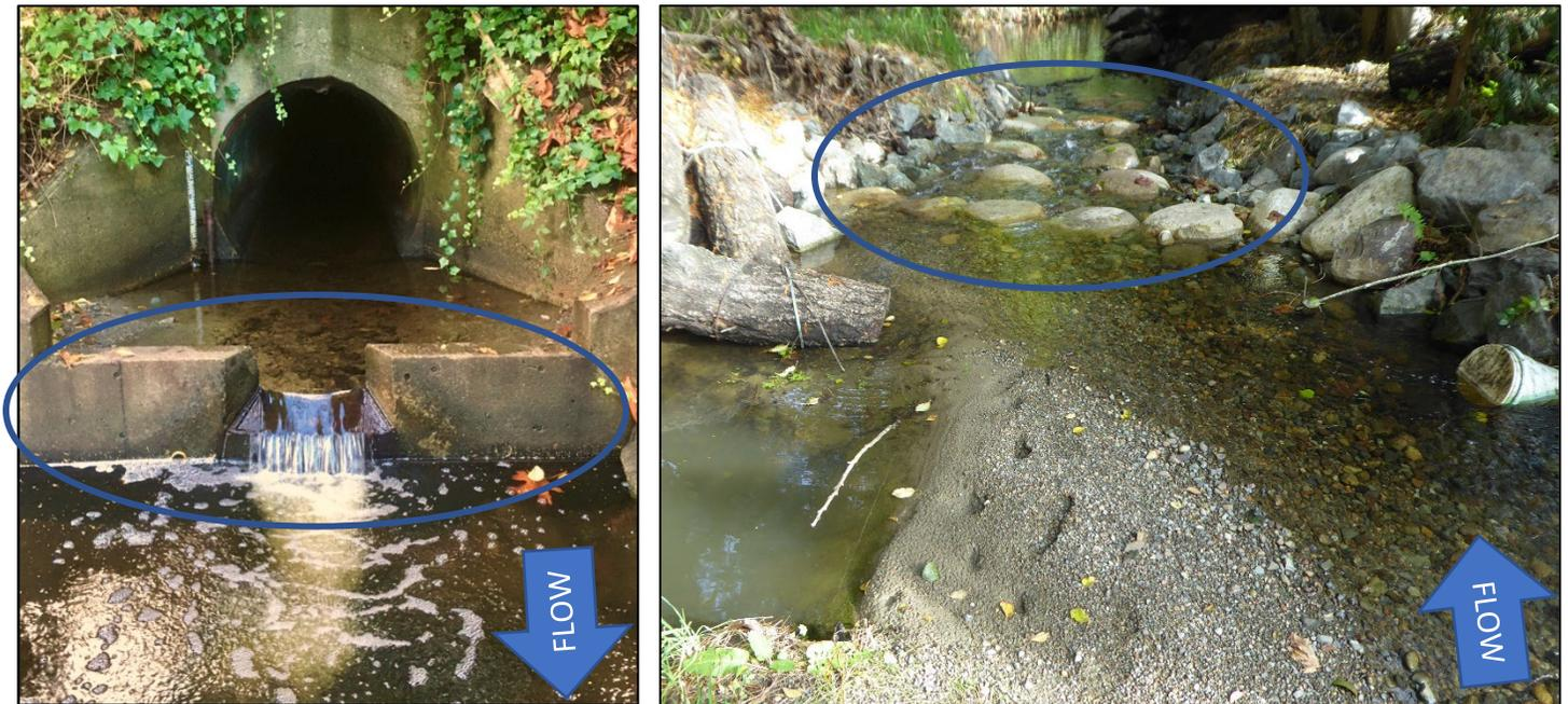
**Figure 2.** Examples of stable artificial controls during low flow.
